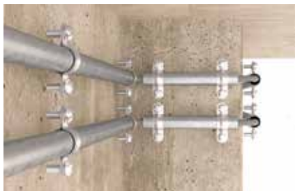
Fixing steel armoured conduits
